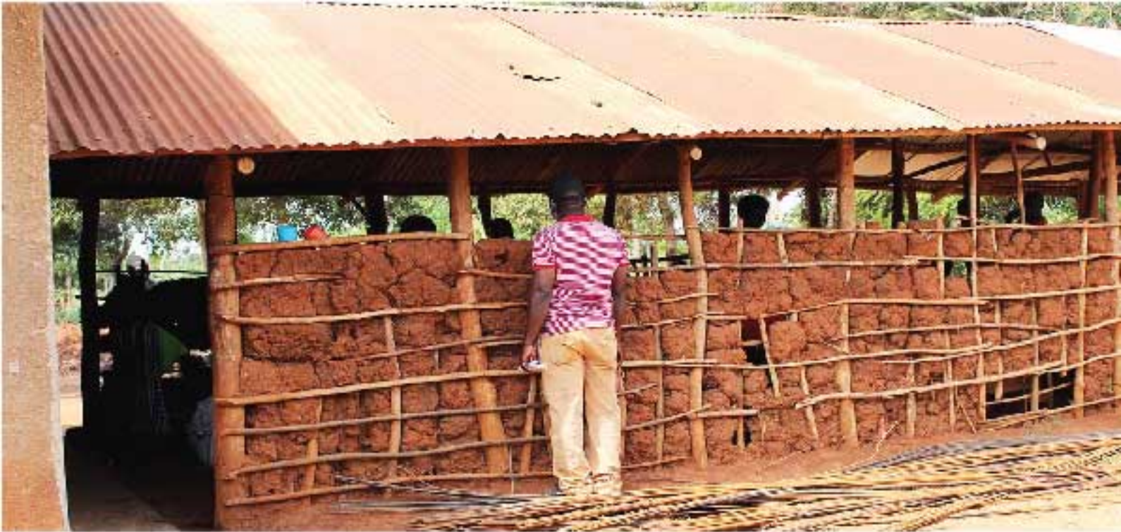
A temporary classroom structure constructed by the parents of Bumeru Primary School
