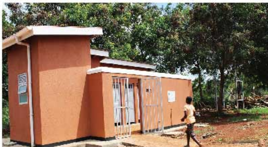
A newly constructed VIP pit latrine at Bumeru Primary School in Mutumba Sub county
