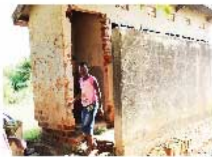
An old pit latrine at Buchumba Primary School
